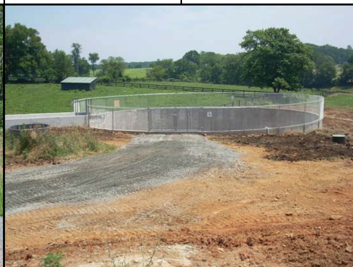
Animal Waste Storage Facility. Dairy waste is stored in this nearly complete concrete structure and then applied to crop fields when the weather is favorable.
