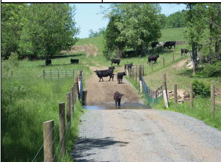
Hardened Stream Crossing for livestock and machinery. Water gates allow water and debris to pass but restrict livestock from moving into the protected riparian buffer.
