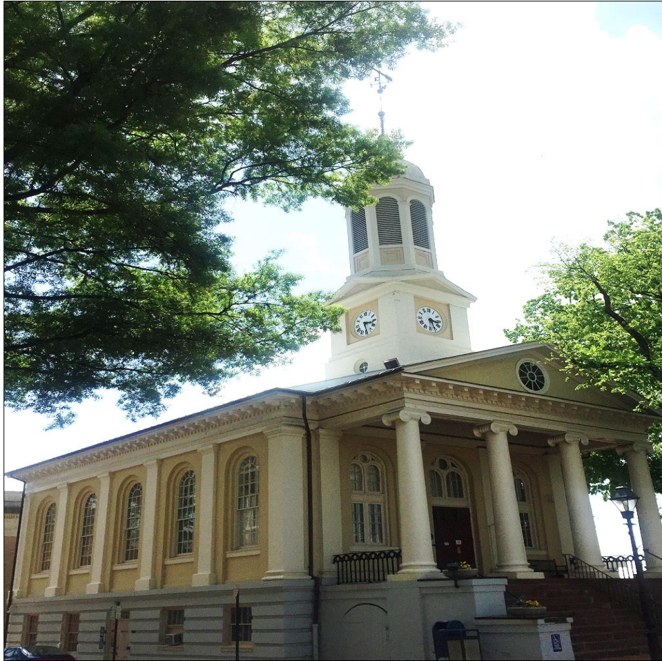
Fauquier County General District Court Warrenton, Virginia
