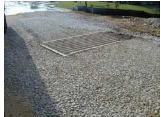
Stone Construction Entrance with Washrack
